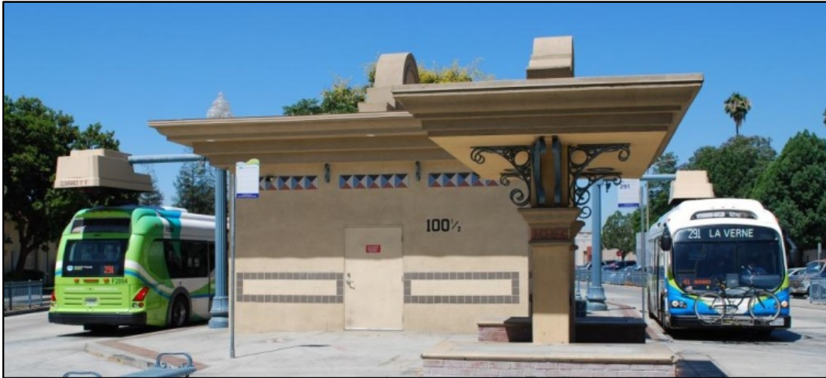
Figure 4. BEB charging station at the PTC
